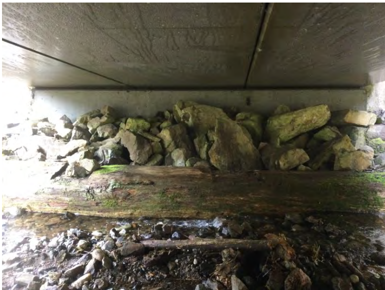
Right Bank Abutment when facing downstream
