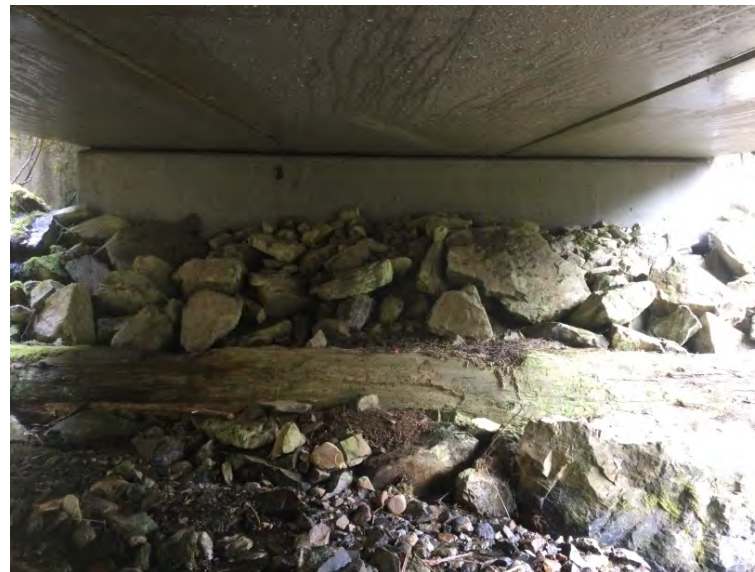
Left Bank Abutment when facing downstream
